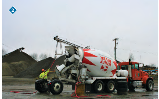
2 Recycled Water Point of Delivery to Delta Sand & Gravel
