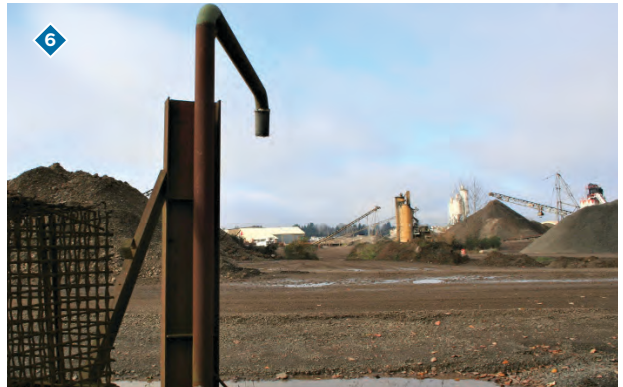
6 Tanker Fill Station
