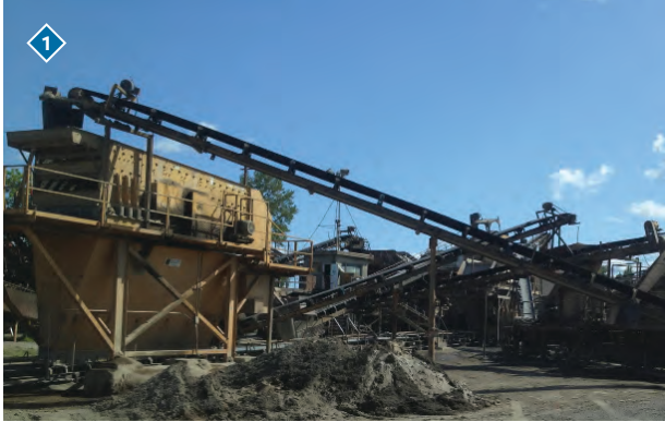
1 West Bank Trail Pipeline Terminus and Metering Location
