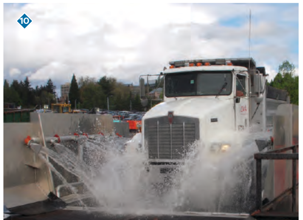
10 Wheel Wash Station CREDIT: Meeds Environmental, LLC
