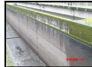
**Description:** In 2023, condition assessment efforts found existing structures needing concrete rehabilitation and other repair work related to primary clarifiers #1 and #3 and the final treatment chlorine contact basins originally constructed in 1980 and 1983, respectively. This project will look for solutions to repair and/or replace existing concrete and other systems related to MWMC past construction contracts C2 (primary treatment) and C6 (final treatment).
